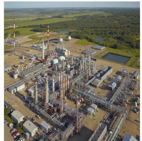
Keyera's Rimbey Gas Plant
