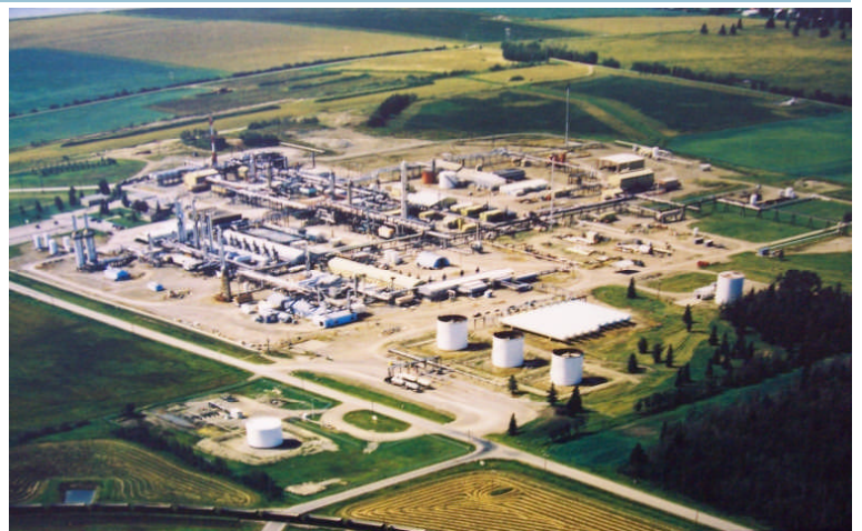
Harmattan Gas Plant
