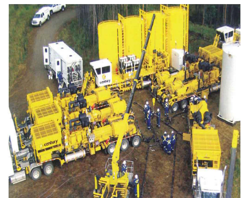
Century Hydraulic Fracturing work-over at a well site in Northern Alberta
